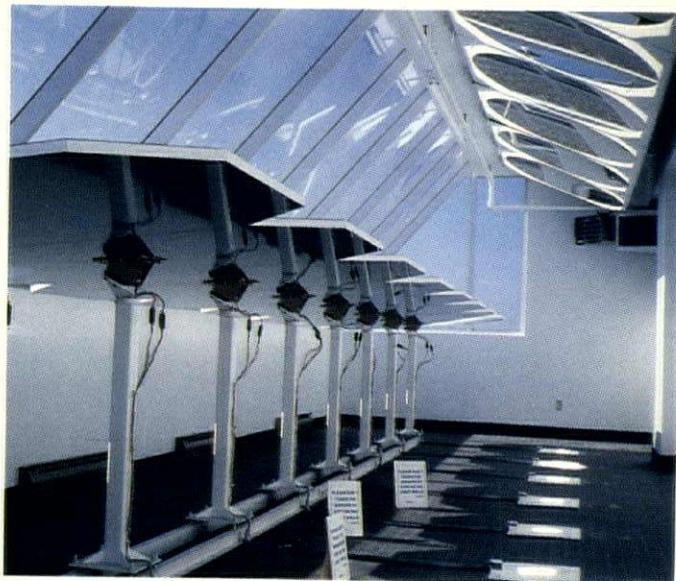
*Solarium with heliostats.*
