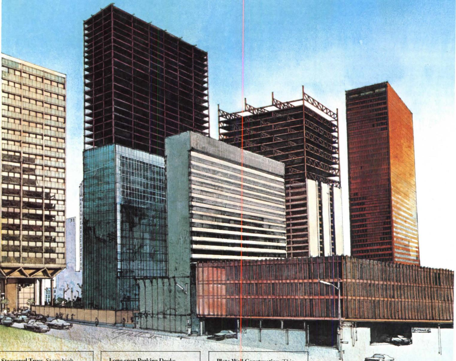
**Staggered Truss.** Story-high trusses that span transversely between exterior steel columns, in a staggered pattern, from floor to floor. Provides column-free interiors with less steel and simpler foundations. Speeds construction and permits earlier occupancy.
