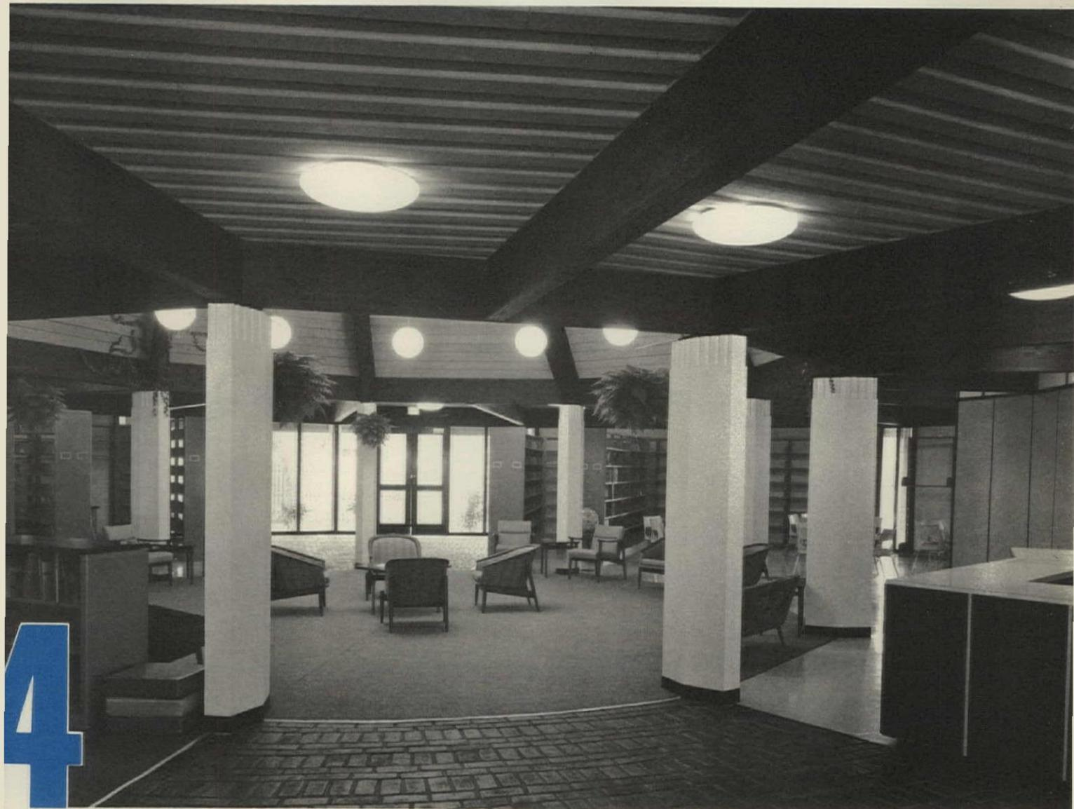
a circular, 40-foot diameter, 18-side building, with exposed laminated Southern Pine beams, Western Red Cedar decking and wall panels.
