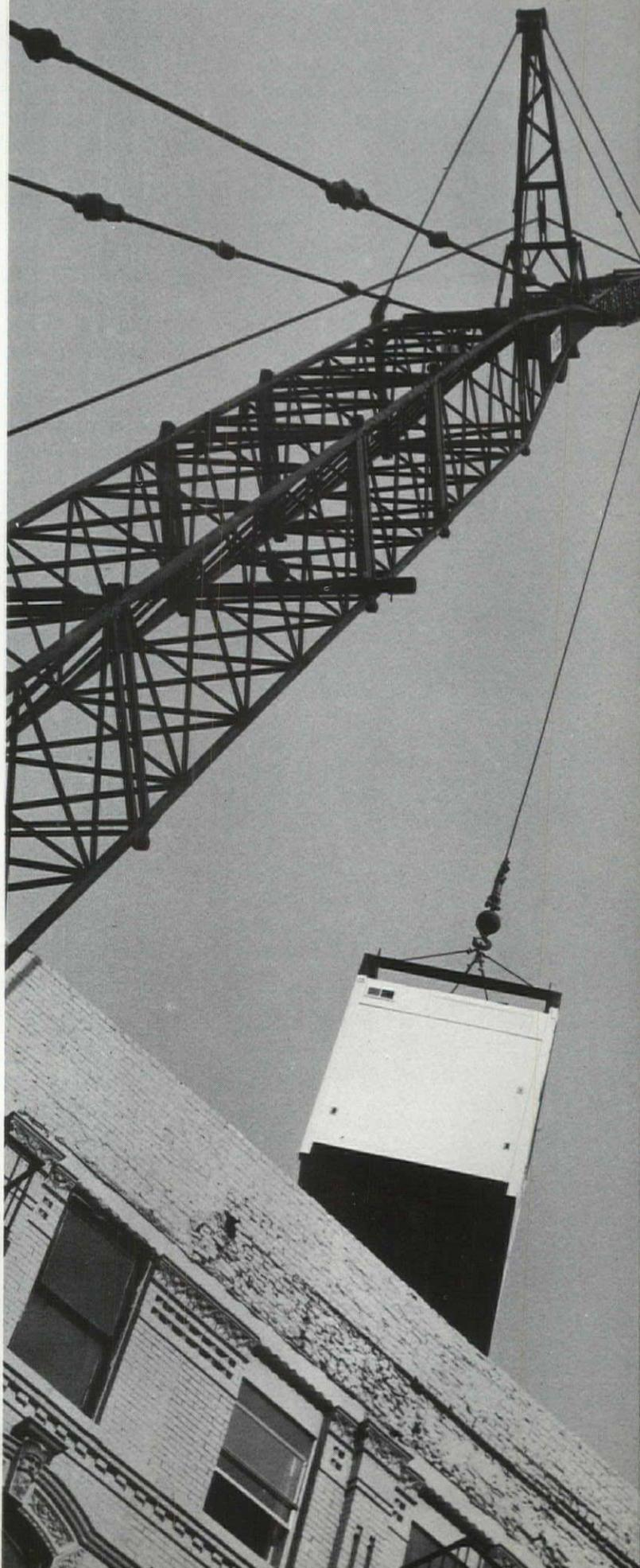
Rehabilitation of a tenement building nears completion in Harlem as workmen (1) prepare brownstone exterior for painting. Aprovingly, a boy (2) catches the show as crane (3) hoists prefabricated core unit containing kitchen and bathroom to workmen (4) atop roof who guide the unit into the hole prepared for it. Lowered into the hole (5), the unit is stacked atop another (6) already in place and ready for use.
