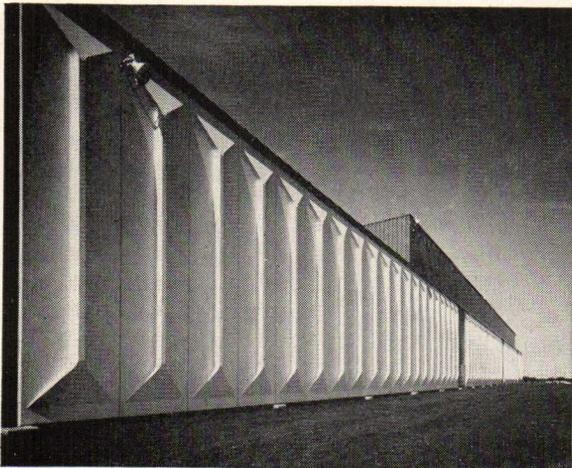
During construction of a new Collins Radio manufacturing plant in Richardson, Texas, the builders put up 162 square feet of exterior and interior walls with every swing of the crane. How? By using pre-cast, contoured white concrete curtain wall panels. Each panel was 6 feet wide by 27 feet high and was made of Trinity White and white marble aggregate.
