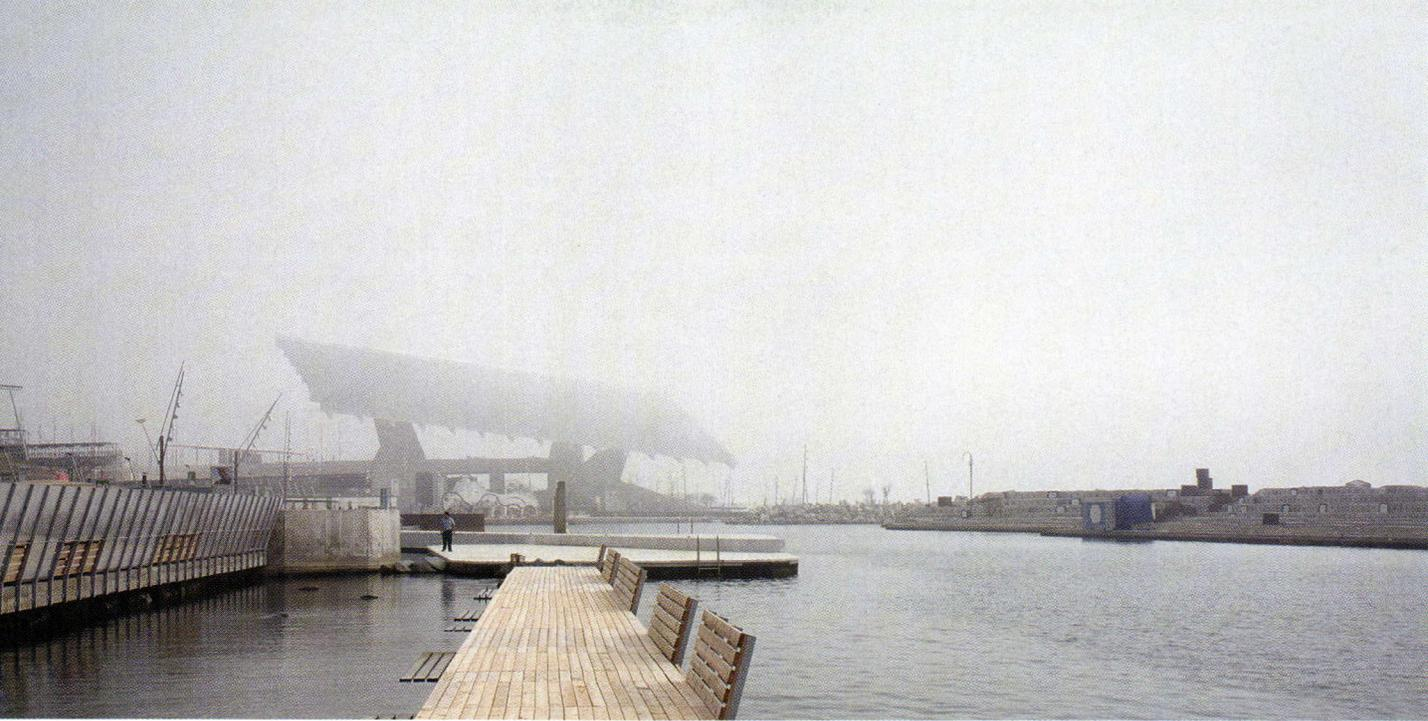
Adjacent to Galí's beachfront is the 113,000-square-foot solar collector (above and below) designed by Elías Torres and José Antonio Martínez Lapeña. Facing south at a 35-degree angle, its 3,700 photovoltaic cells can generate 1.3 megawatts of power.
