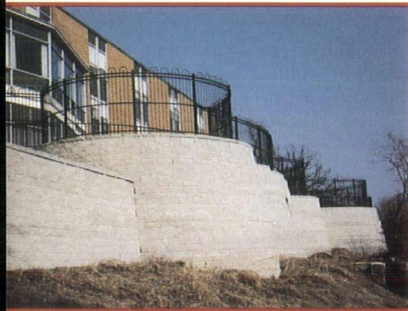
Concave curves built with tight vertical joints.
