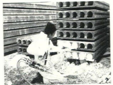
Foaming cores of Spancrete lightweight precast wall panels.
