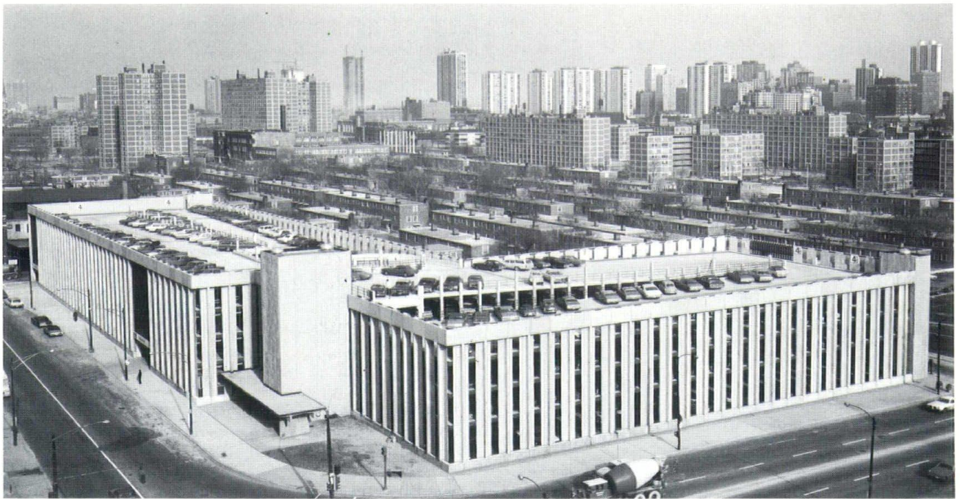
CORPORATE PARKING STRUCTURE: Montgomery Ward & Co., Chicago, Illinois
