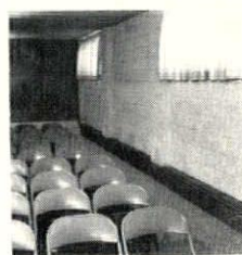
Electric baseboard units heat the basement
