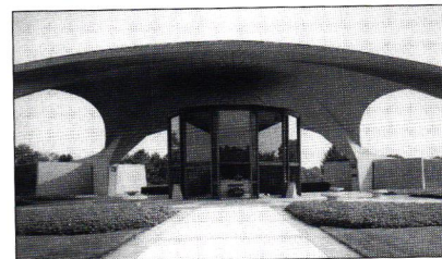
St. Lazarus Oratory is one of the largest clear span post-tension concrete structures in the tri-state area, requiring the special skills of John Deklewa & Sons, Inc..
