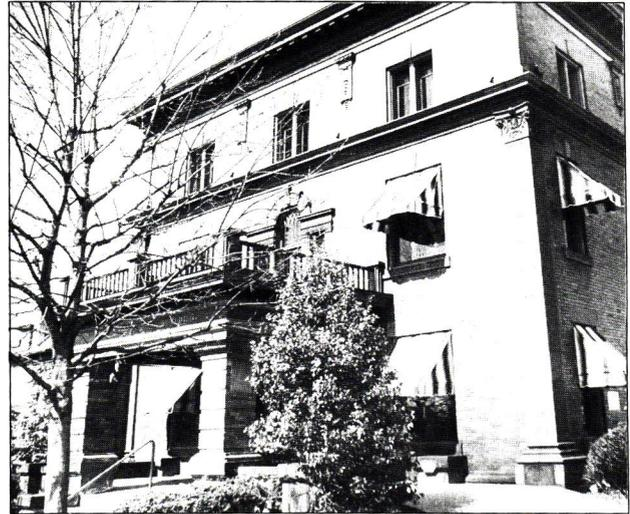
**Above:** The former Troutman mansion, built in 1907, has served as Butler City Hall since 1930. N. Lee Ligo and Associates renovated the interior with a new elevator, sprinkler and alarm systems, wiring and central air; exterior work included reinstallation of the front porch, using old photographs as references.
