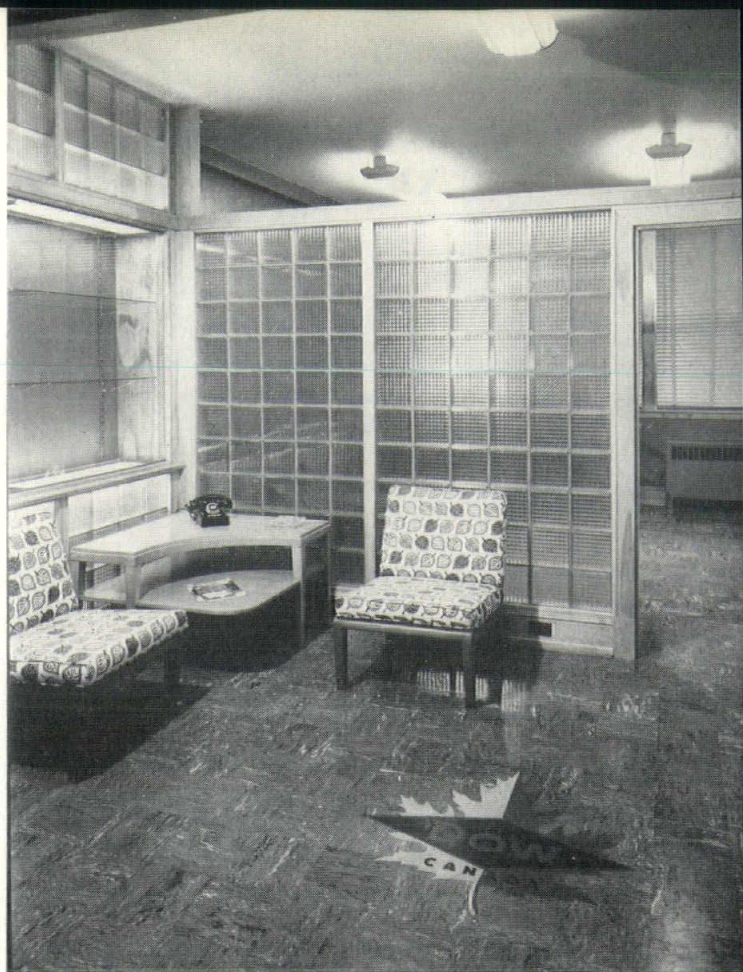
Since office layouts change continually, Bloxolite is particularly suitable as it may be dismantled and erected again with the same materials.
