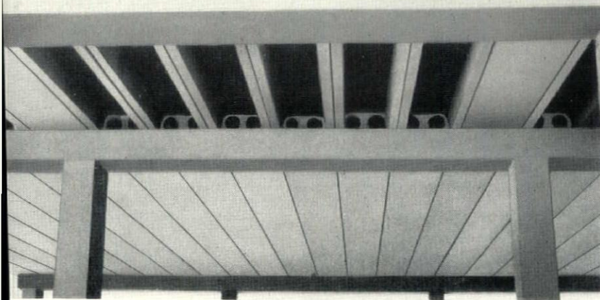
Some of the many advantages of the new structural system with FLEXICORE are shown in these photos. Built-in wiring raceways in roof are easily accessible.
