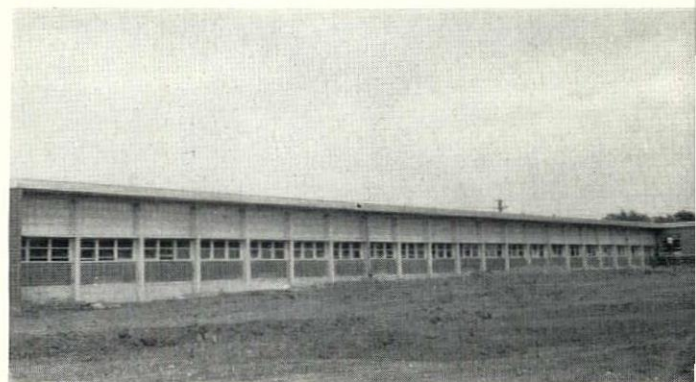
Roof forms overhang to make sun shield. Exterior gives strong, sturdy appearance, reflects high-quality construction, yet precast materials make cost low.
