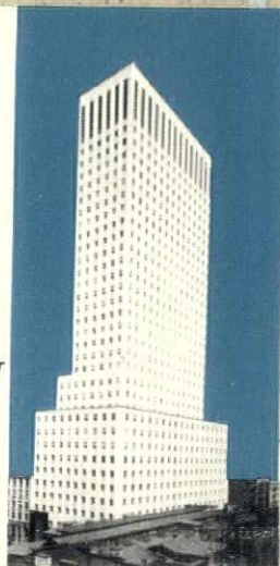
East Building, New York City Architects: Hofmeister and Falquist Hanley Duramic No. 824 Limestone Grey with medium speck
