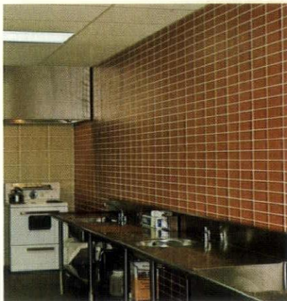
Flexible scale in acid and alkali resistant walls.
