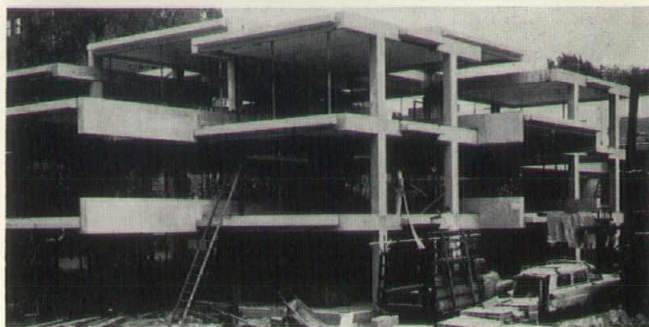
TOP: Model shows structural framework of precast concrete units. ABOVE: Construction is shown well under way as framework is nearly completed. BELOW: Precast beam with lugs for support of hollow precast prestressed concrete floor planks is being lowered into place. BOTTOM: Detail of corner in the structure shows joint line between precast units.
