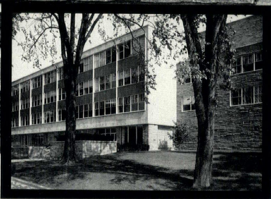
Phillips Hall—Cornell University, Ithaca, N. Y. Architects—Perkins and Will, Chicago, Ill. Contractor—White General Construction Co., Inc., New York City LENROC SAWED—BED ASHLAR
