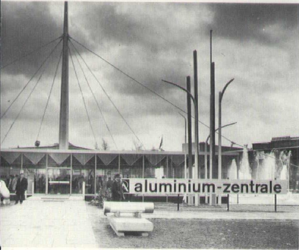
The roof assembly, the top surface of which is flat, is supported from above by a series of tension cables radiating from the top of the aluminum mast.
