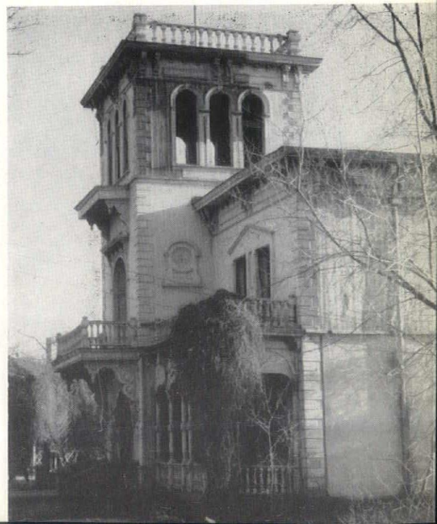
fig. 2—exterior: entrance and front porch
