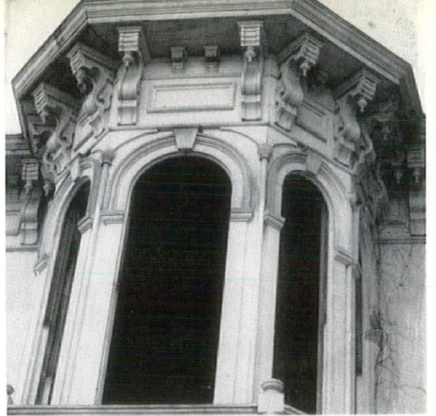
fig. 6—exterior: front bay window detail
