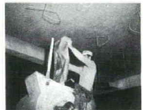
2 Finished fireproofing treat- ment presents pleasing sur- face and texture. Photos tak- en at Bell Telephone Co. Building, Pittsburgh, Pa.
