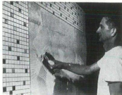
No special preparation of back-up needed. Here TILE-SET is floated on dry portland cement brown coat. Special notched trowel gives proper thin-bed mortar thickness.
