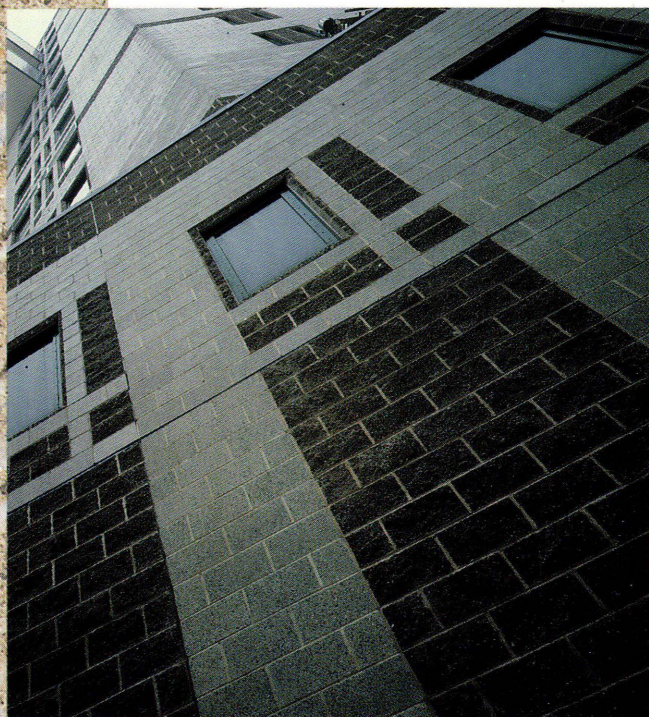
The new Union County Correctional Facility is supported by 130,000 units of Anchor Ground Face Block and 30,000 units of Anchor Split Face Block.
