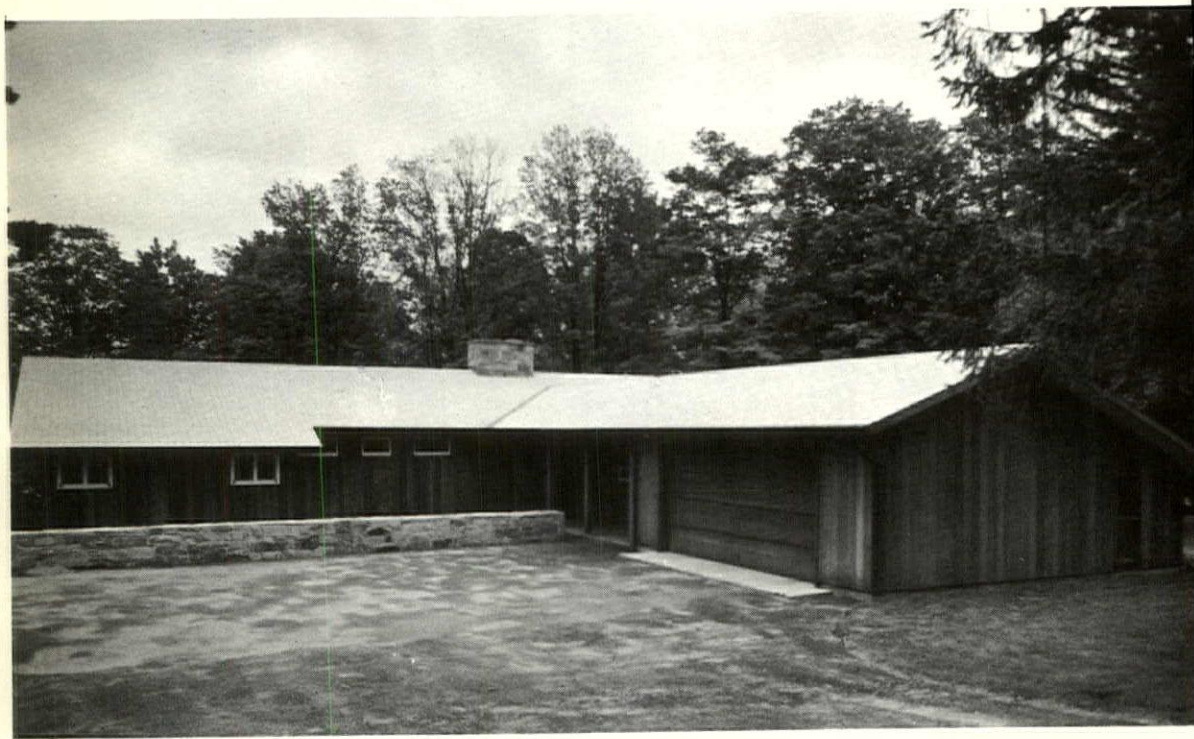
Entrance Court: privacy within is provided by very limited window area on the "public" side of the house, contrasted to the fully open "private" side shown in photo #1. Traffic is subtly directed to the front door by the low stone wall which also keeps vehicles away from the house itself.
