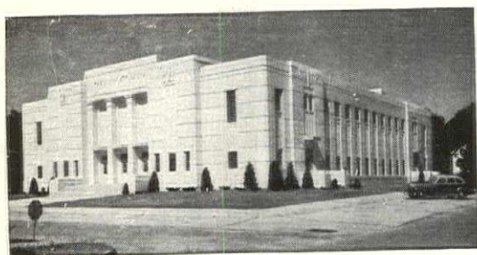
City Auditorium, York, Neb., designed by Meginnis & Schaumborg, architects, of Lincoln. Architectural concrete details produced by use of milled wood and plaster molds. Smooth exterior concrete walls cast in plywood forms.
