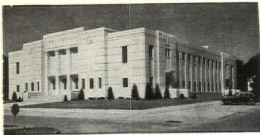
City Auditorium, York, Neb., designed by Meginnis & Schaumburg, architects, of Lincoln. Architectural concrete details produced by use of milled wood and plaster molds. Smooth exterior concrete walls cast in plywood forms.
