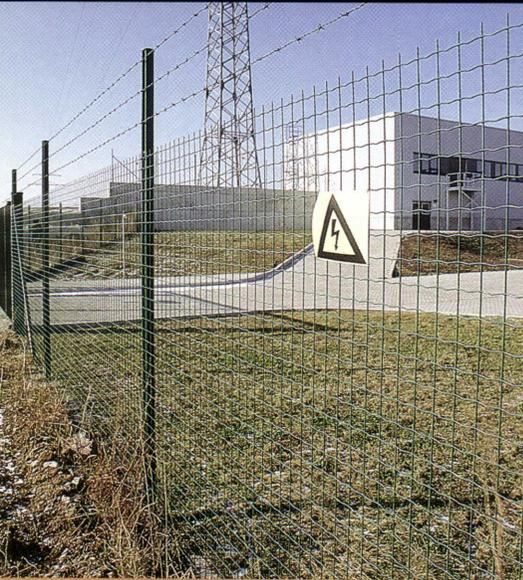
*Fortinet Medium, with its 2-inch square welded mesh, meets the strict security regulations for fencing surrounding this electrical facility.*
