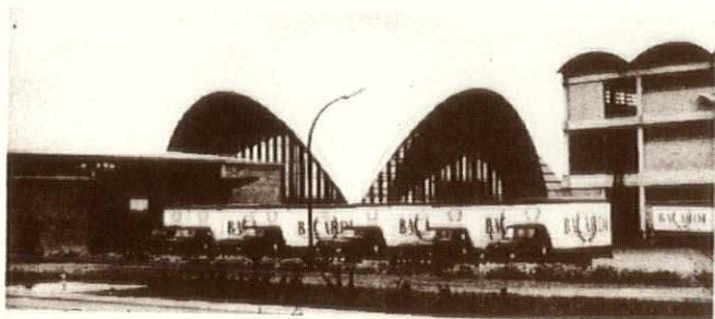
ABOVE:—Shells like this one erected at a new Bacardi bottling plant outside Mexico City are becoming a fairly common sight in the U.S. Inside the plant the interior was left plain, and unfinished.
