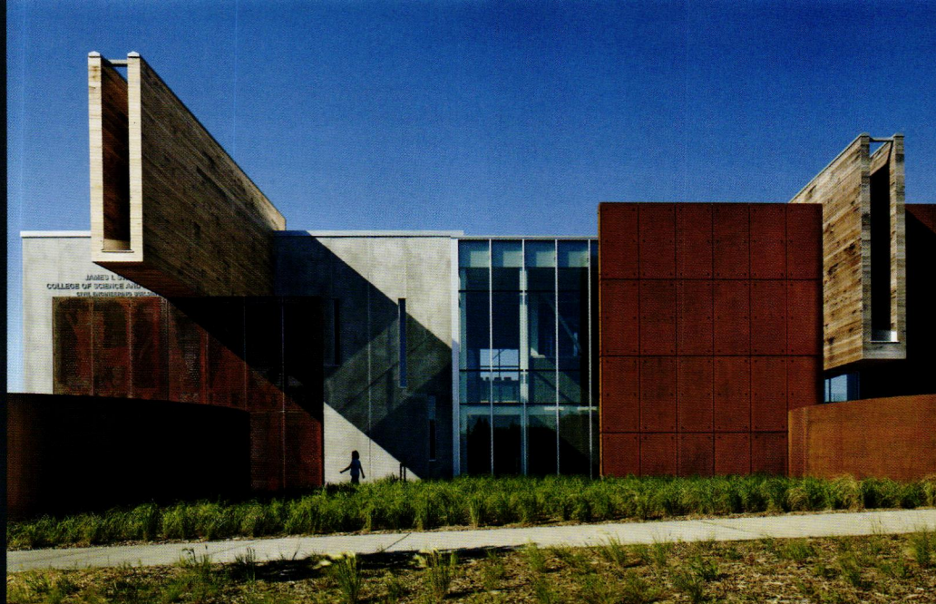
Left: Giant reclaimed wood scuppers divert stormwater to a drain system for filtration and reuse. Below: The structural and hydraulic labs accommodate two 15-ton gantry cranes. Bottom: An 11-ton bifold door enables access for large structures and equipment.
