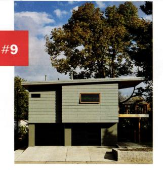
The ADU's canted roof extends over the secondfloor deck. The garage ceiling was lowered to maximize the height of the living space above.
