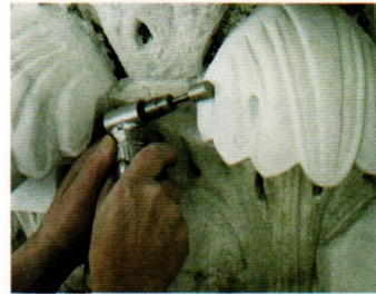
One of the many stonemasons on the project blends a Dutchman replacement into one of the building's many capitals.
