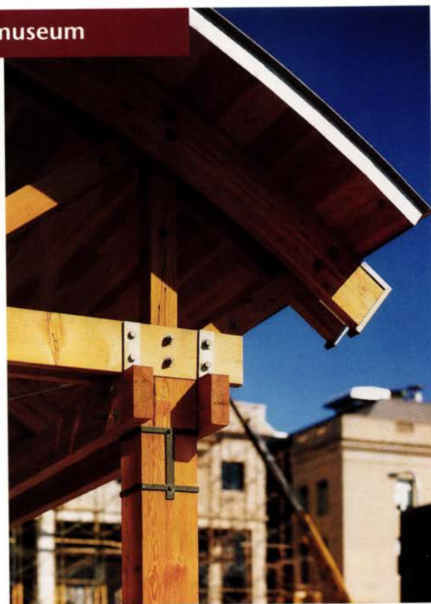
The architects reused such material as heavy timber gutted from the interior to fashion an entrance canopy (above and opposite) for the converted industrial building. The modern core juts above the roof line (top).
