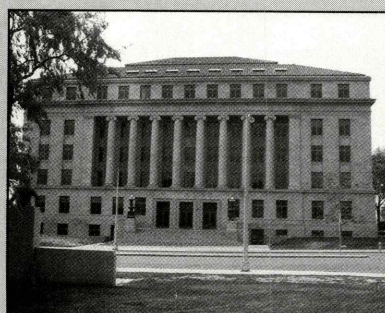
State Office Building, St. Paul Complete window replacement.
