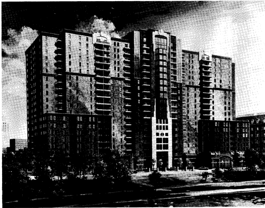
The 23-story Riverwest apartment complex, designed by Korsunsky Krank Erickson
