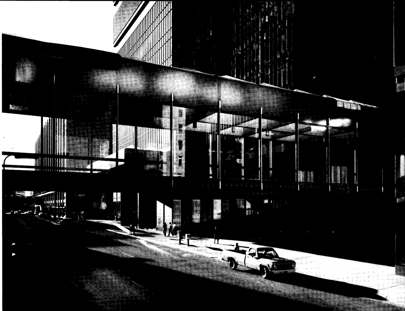
The IDS skyways: they echo the building's design
