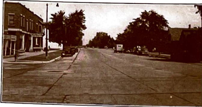
CURB AND GUTTER, ROCHESTER, MINN.
