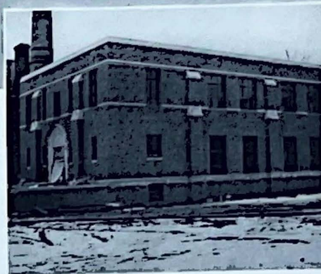
Power Plant, Hamline University, St. Paul
