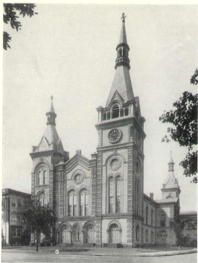
Dwight Place Church, New Haven, Conn., built entirely of precast concrete in 1871 and still in regular use establishes cast stone as an "old" material.
