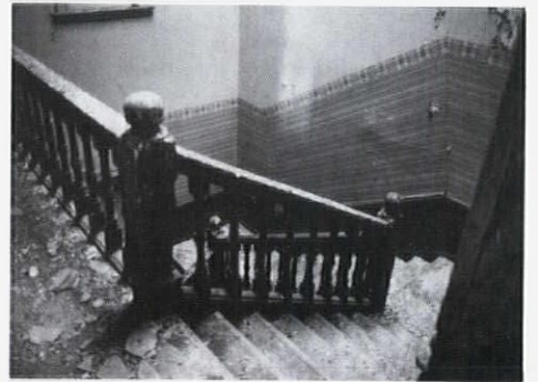
Due to extensive water damage, reconstruction of portions of the interior was necessary, including the stairwell which was rebuilt using original newel posts.
