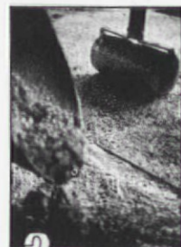
2 Placing and compacting TERRAZZO topping.
