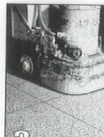
3 Grinding and finishing TERRAZZO floor.
