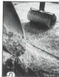
2 Placing and compacting TERRAZZO topping.
