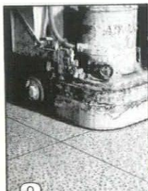
3 Grinding and finishing TERRAZZO floor.
