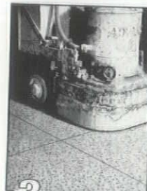
3 Grinding and finishing TERRAZZO floor.
