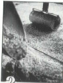
2 Placing and compacting TERRAZZO topping.
