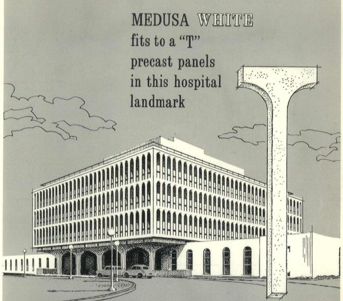
The entire exterior facade (23,000 sq. ft.) of this striking hilltop hospital is composed of approximately one thousand white precast units with glistening white quartz aggregate.
