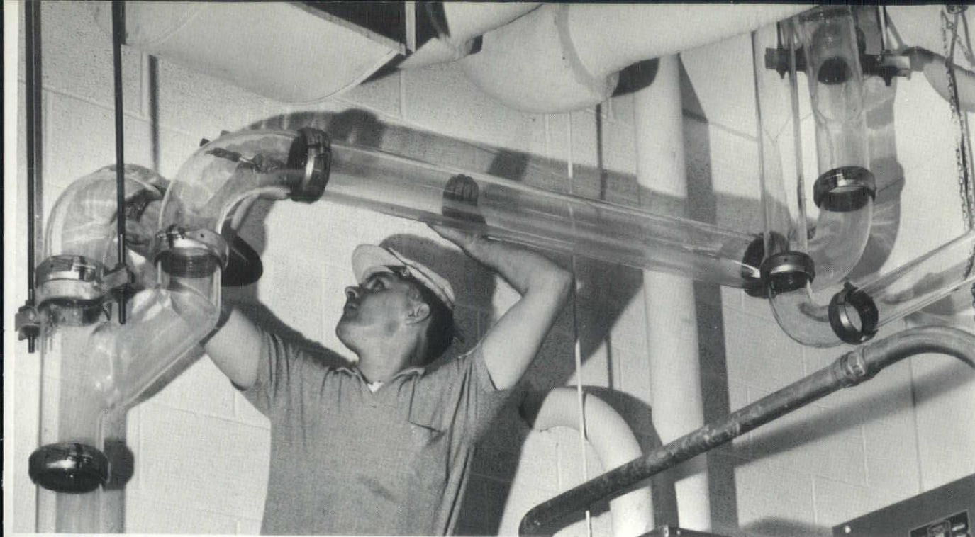
See through pipe. Coming into more wide-spread usage, for many applications, is glass pipe. It has been found to be near ideal in meeting certain laboratory and chemical handling specifications.
