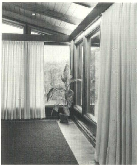
Low velocity conditioned air is distributed at the floor perimeter by Smooth-Aire diffusers. Dimmer controlled lighting is concealed behind valances above the windows.
