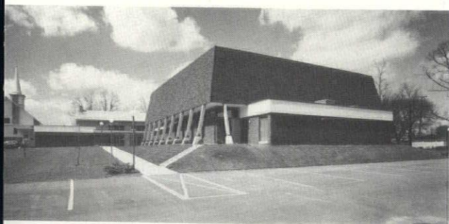
The Cascade Christian Church, designed by OBryon and Nachtegall, Inc. Architects, Grand Rapids, Michigan. Plywood framing system was fabricated and erected by Roof Structures Inc. Webster Groves, Missouri and the general contractor for the job was Boersma Builders, Grand Rapids, Michigan. Stress skin panels were prefabricated under cover utilizing economies in both construction and erection. Photo by Bernie Photographs
