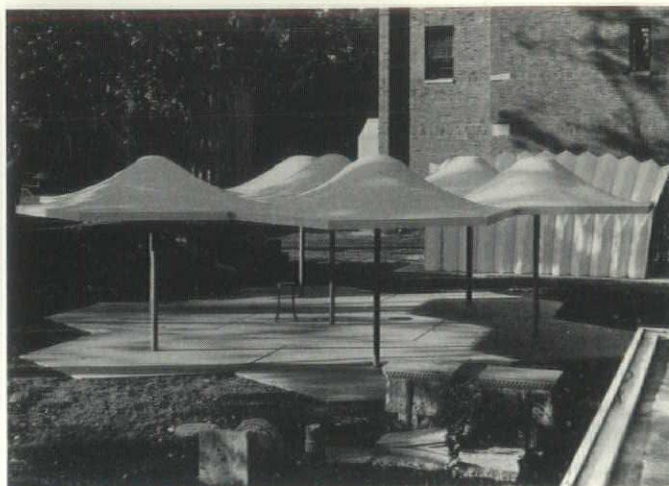
Completed pavilion structure constructed of anticlastic membrane umbrella shell components.
