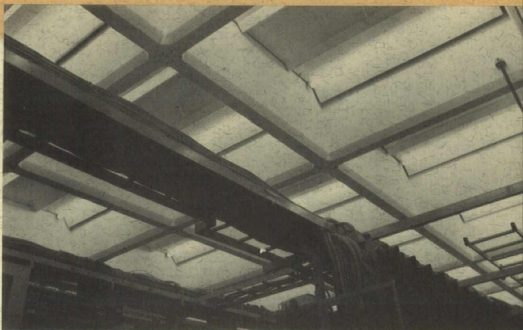
Ceiling illumination in the communications center presents a busy pattern. Condensation and integration of structural, architectural, mechanical and electrical elements resulted in a ceiling to floor construction depth of 3' 1", providing luminous ceilings and air distribution normally requiring upwards of 4' 10".
