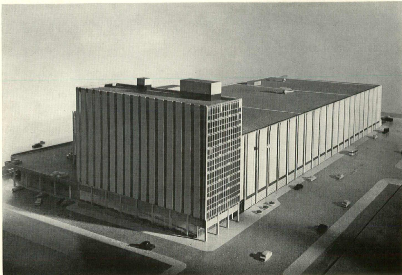
DETROIT'S NEW POST OFFICE GIFFELS AND ROSSETTI, ARCHITECTS AND ENGINEERS BARTON-MALOW COMPANY, GENERAL CONTRACTORS FLEXICORE, EIGHT FLOORS 75,000 SQUARE FEET, ELECTRIFIED PRE-CAST WALL PANELS, 27,000 SQUARE FEET
