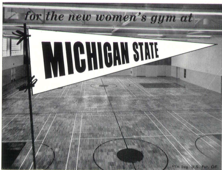
18,600 sq. ft. 33/32" Edge-Grain Ironbound Floor in Women's Gym, Michigan State U., East Lansing, Mich. Arch.: Ralph R. Calder, Detroit, Gen'l Contr.: Granger Bros., Lansing. Installer: Bauer-Foster Floors, Inc., Detroit.
