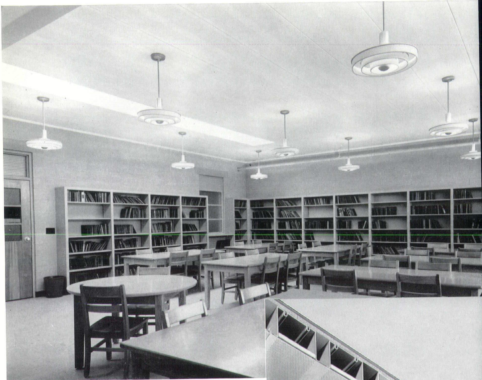
M-Deck Acoustical Ceiling in the Library of the Bonlee-Goldston Consolidated High School recently constructed for the Board of Education, Chatham County, North Carolina. The school has Sixteen Classrooms, an Auditorium, Cafeteria and Shop in four buildings. Mahon Long Span M-Deck provides the Roof Structure and Finished Ceilings for the entire project, including covered, connecting walkways. Architects: Simpson & Savage. General Contractor: Hunt Construction Company.
