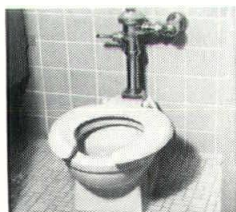
Briggs Tot Water Closets, vitreous china syphon-action models, 10" high, used in the Academy kindergarten.
