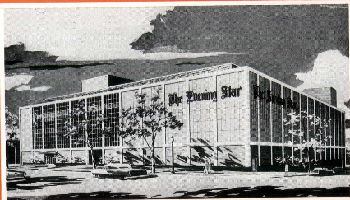
NEW BUILDING for Washington Star achieves interesting curtain wall effect with colored Marietta precast panels framed by white horizontal and vertical trim. Faulkner, Kingsbury & Stenhouse, Washington, D.C., architects; Gongwer, Krass and Webb, Washington, D.C., structural engineers; Charles S. Leopold Engineers, Inc., Philadelphia, Pa., mechanical engineers. The Charles H. Tompkins Co., Washington, D.C., general contractor.
