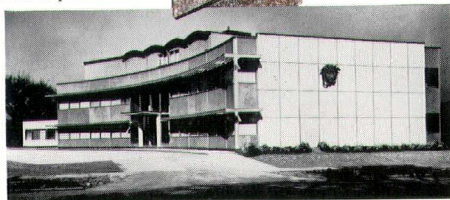
MARIETTA WALL PANELS in headquarters building for Medusa Portland Cement Co., Cleveland Heights, Ohio, are suspended from cantilevered lift-slab floors. No grid supports are used. Ernest Payer, A.I.A., architect; Brown Construction Company, general contractor.
